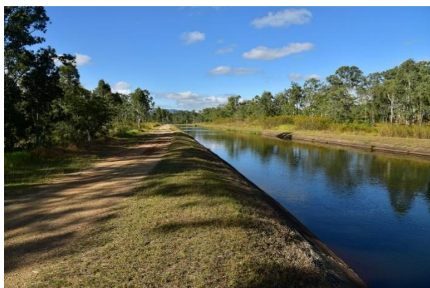
Figure 5. West Barron Main Channel. Photo: K. Martin.
